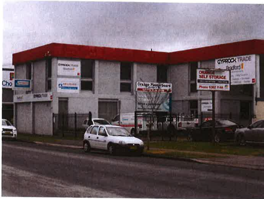
Plasterboard warehouse opposite in Dalton Street
